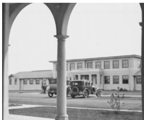
The old Jolimont building, Alinga Street, Canberra, 1929
