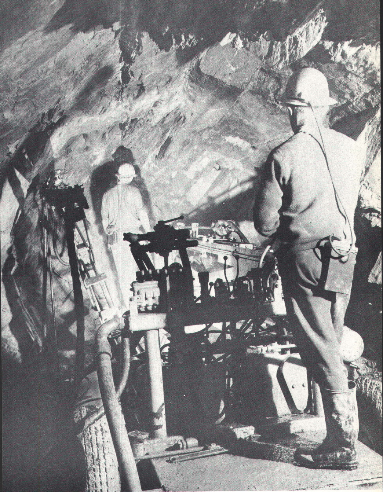
Hard-rock miners drilling a drive face at the Rosebery Mine
