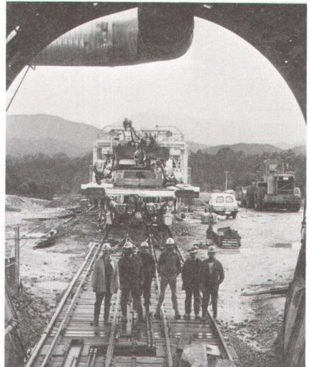
Jumbo drill, weighing 85 tonnes and costing \$1.2 m, used on the King headrace tunnel.
