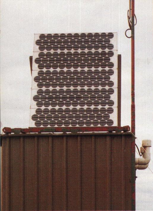
*A solar collector is used to power the radio base station at Mt. Huxley.
