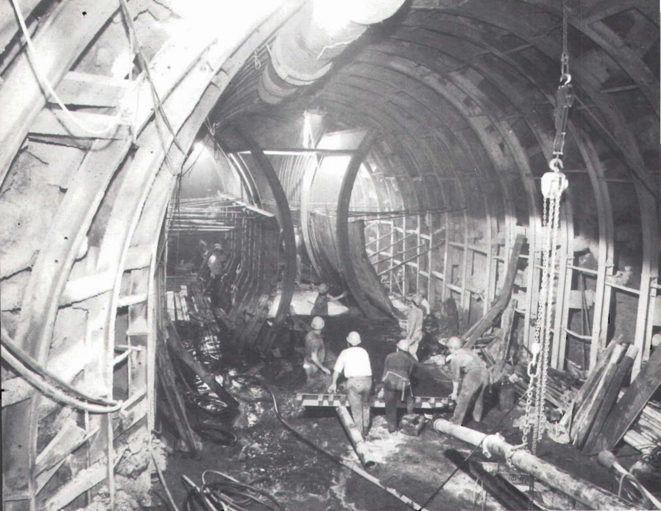
An Alpine mining machine is used to excavate the foundations for the Flagstaff Station site—part of Melbourne's new underground railway.
