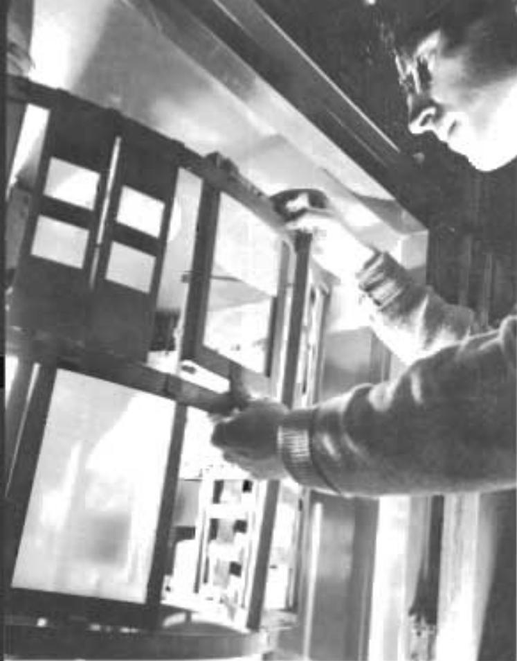
Accelerated weathering tests on plastics, dyestuffs, and pigments are carried out at research laboratories at Ascot Vale.
