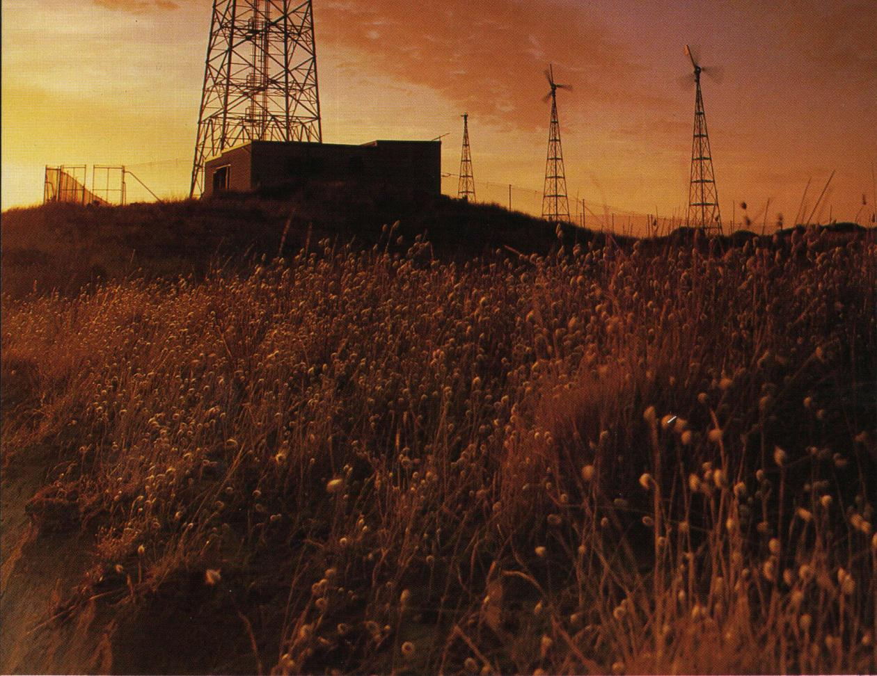
*Cape Wickham microwave repeater on King Island, Tasmania showing the wind generators which provide power for the telecommunications equipment. (Telecom Australia)*
