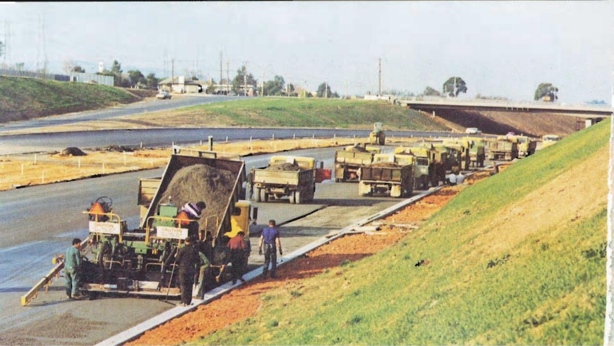
Asphalt sealing in progress on the Mulgrave Freeway, July 1976.
