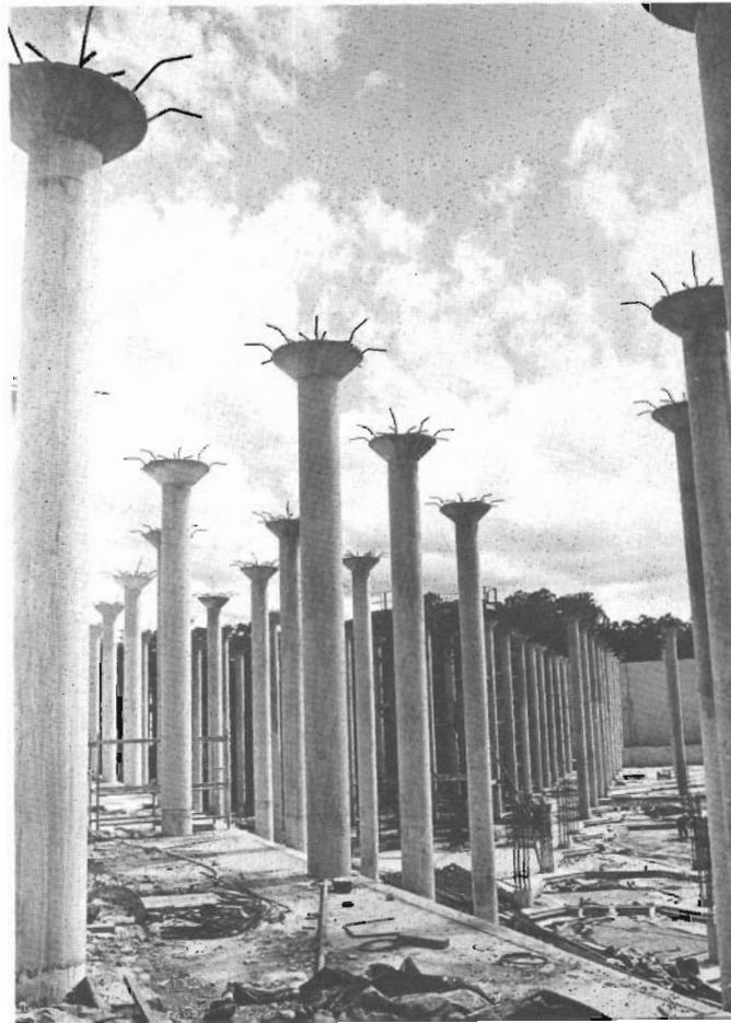
Support columns for the roof of the Sugarloaf Reservoir clear the water storage which will have a capacity of 200 megalitres.
