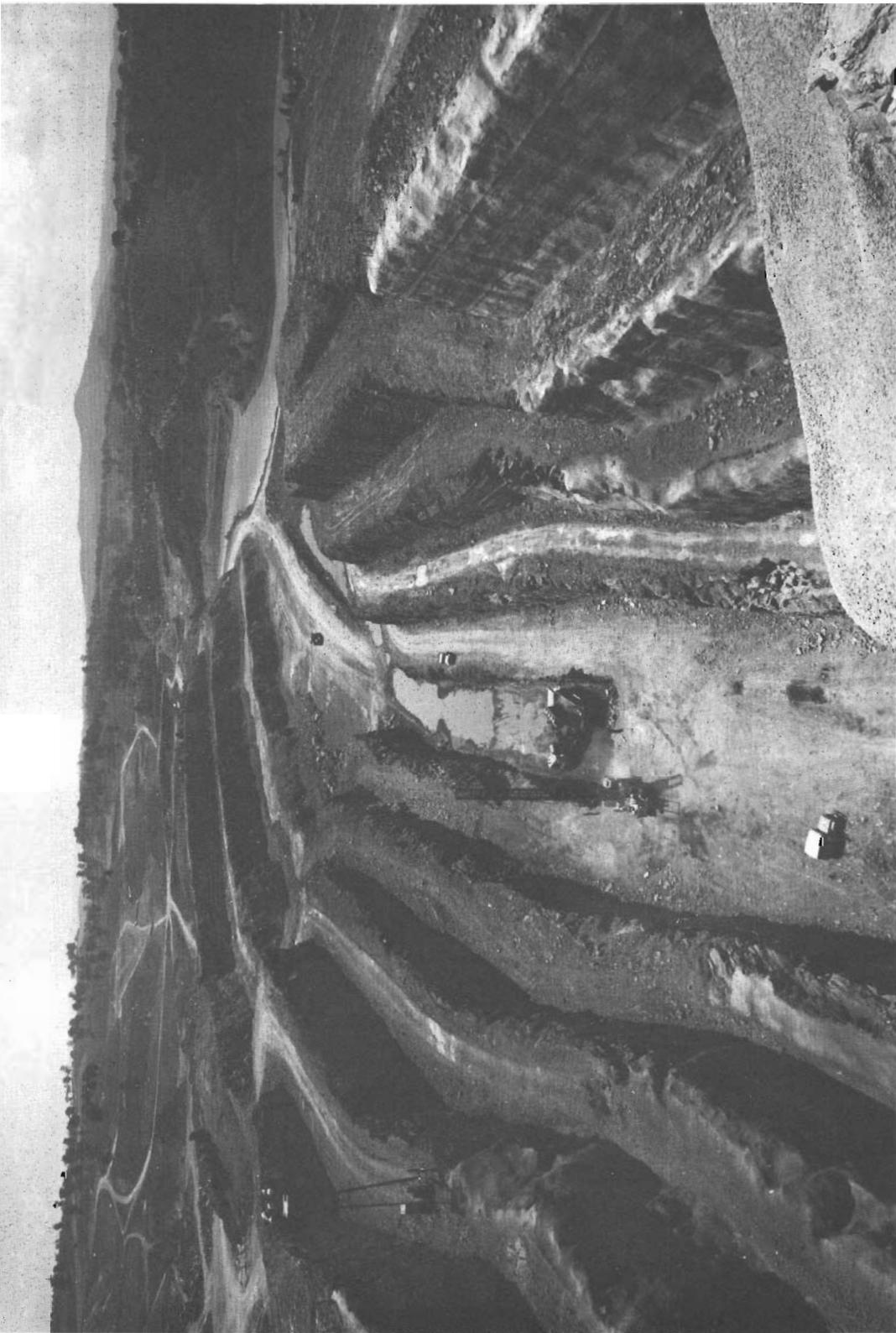
Excavation for the draw-off channel which will convey water from the Sugarloaf Reservoir in the Christmas Hills area for delivery to the water treatment plant.
