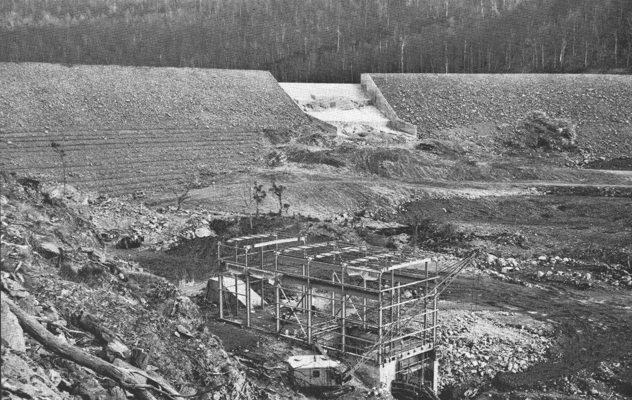
Rowallan Dam with power station under construction
