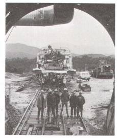
Jumbo drill, weighing 85 tonnes and costing \$1.2 m, used on the King headrace tunnel. Photo: Advocate
